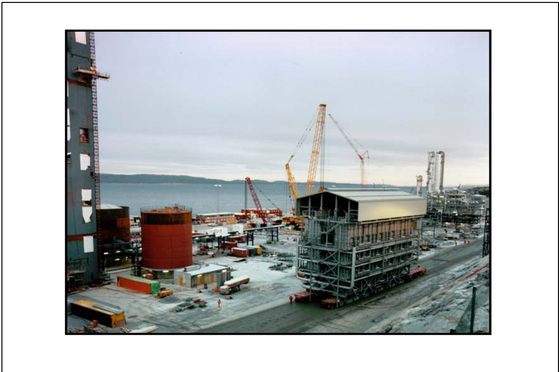
Photos: View of Tubular Reformer under Transport at Site
