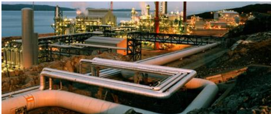
Statoil industrial complex at Tjeldbergodden
